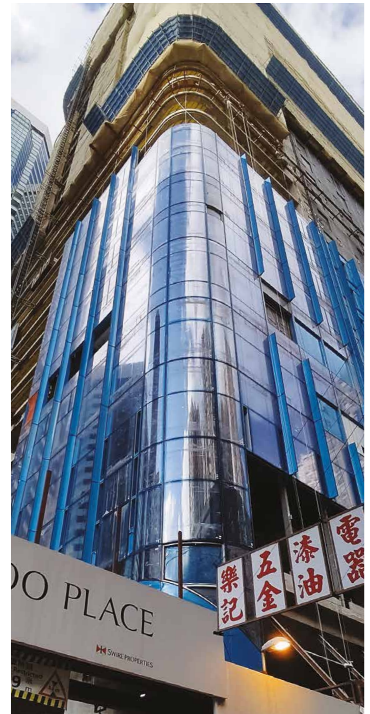
Two Taikoo Place Installation of the glazed curtain wall
