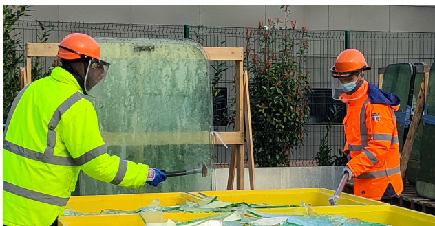
Top left: Unesco in Paris forms a pilot circular project of cladding reuse and glass recycling
